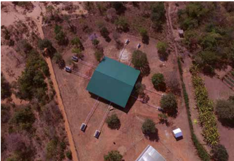
Aerial picture of the flight cage (green roof) surrounded by 8 tents. Air-conditioning ducting brings odor from the tents into the cage
